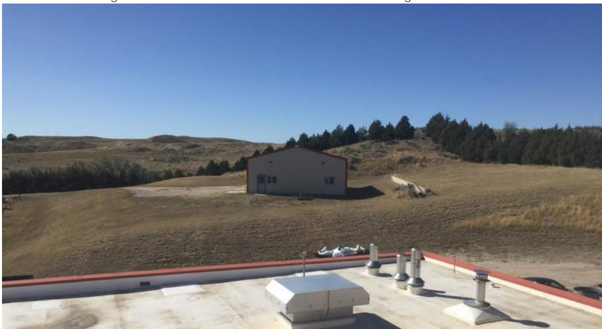
Maintenance Building as Viewed from the Roof of the Main Building
