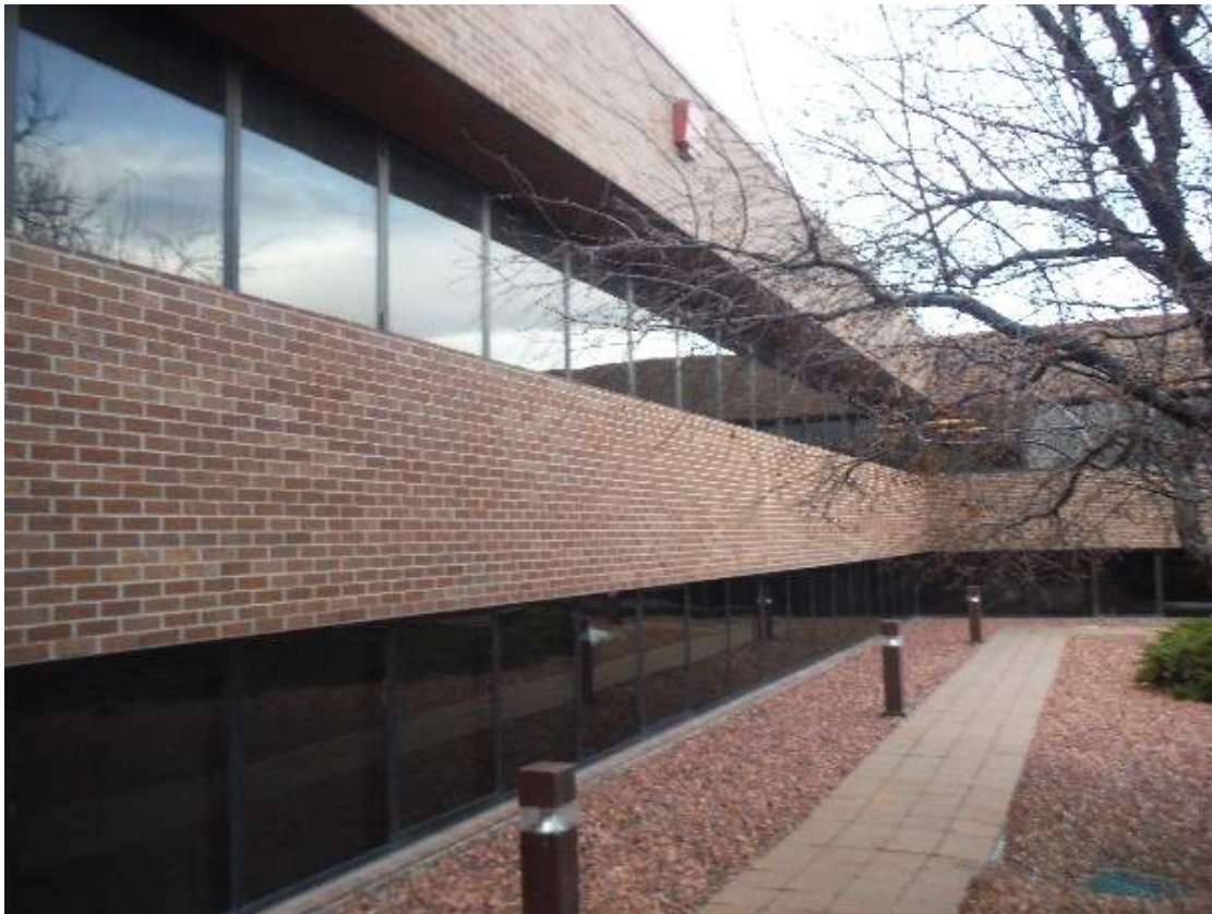
Photo 1 - Area A in Courtyard
