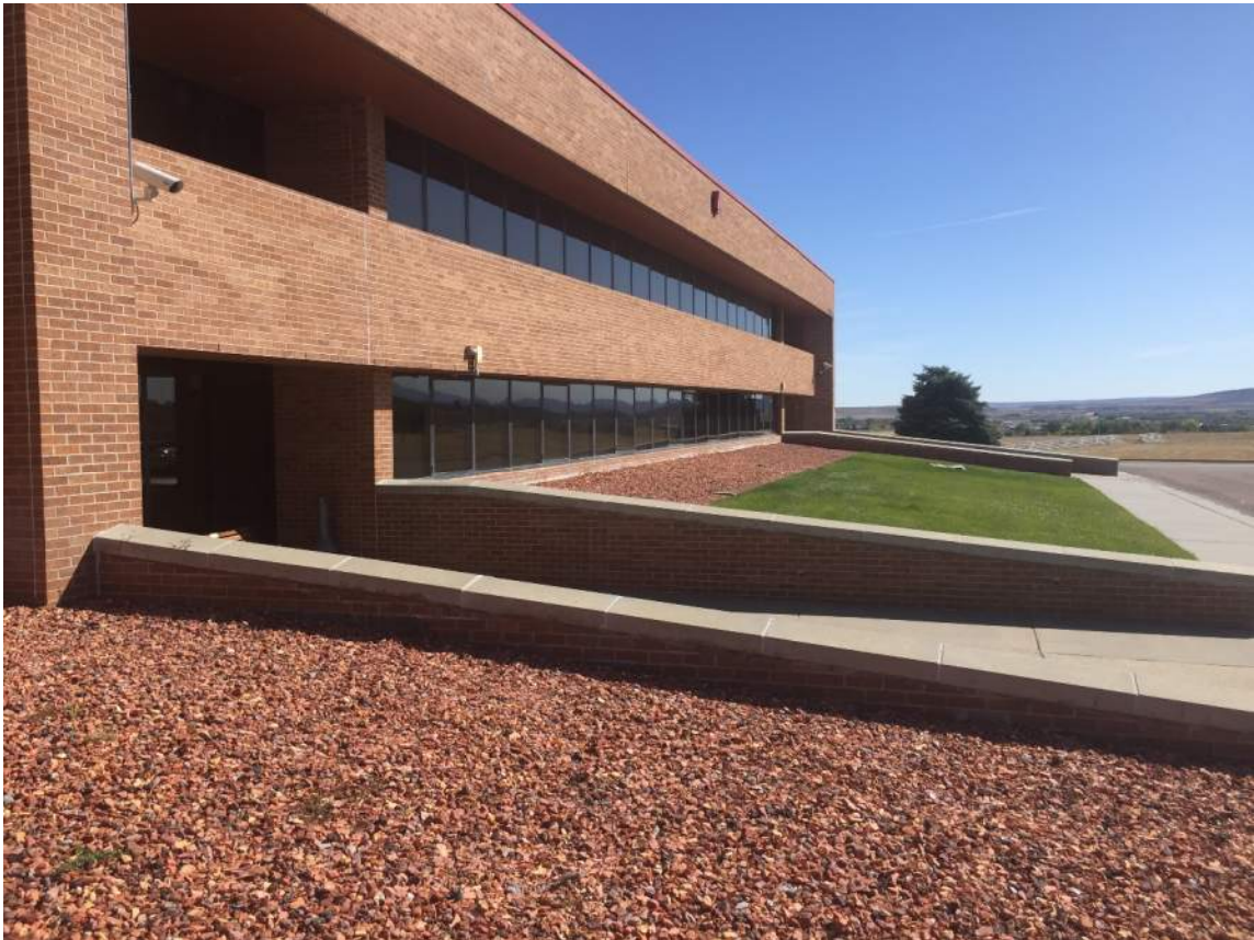
Existing Dormitory Facility – Exterior Entry View
