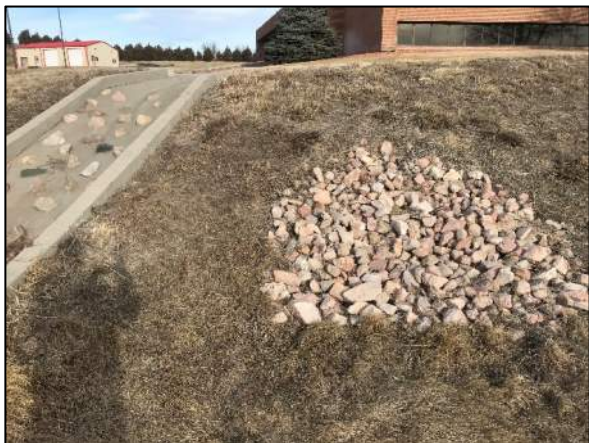
Drain Outlet & Curb Cut Near Southwest Corner of WLEA
