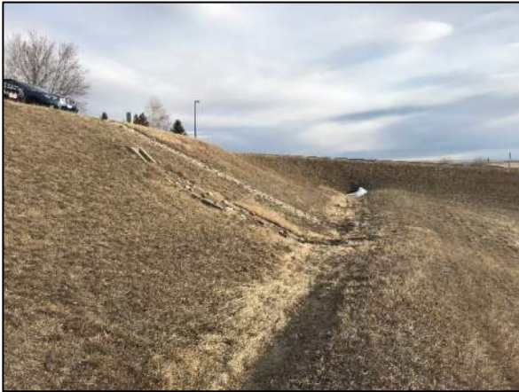
Drainage Channel South of Visitor Parking
