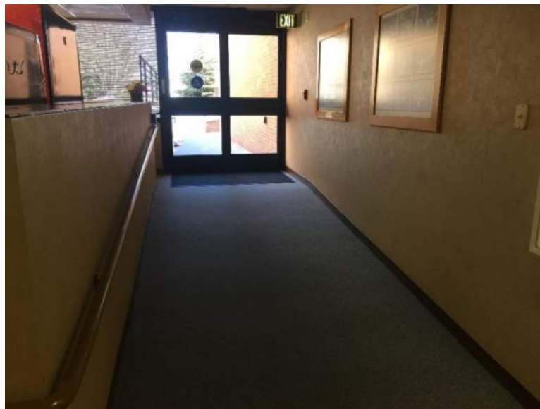
Double Aluminum Doors w/ Operator at East Courtyard Entrance
