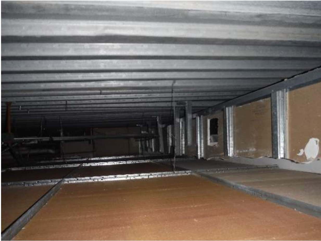
Area A – Framing at Corridor Ceiling Plenum
