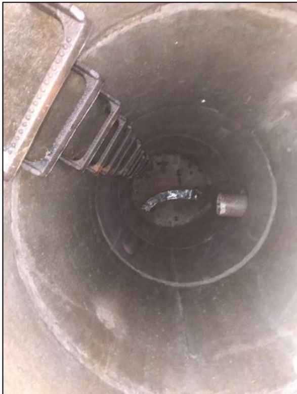
Drop Manhole Near Road Crossing
