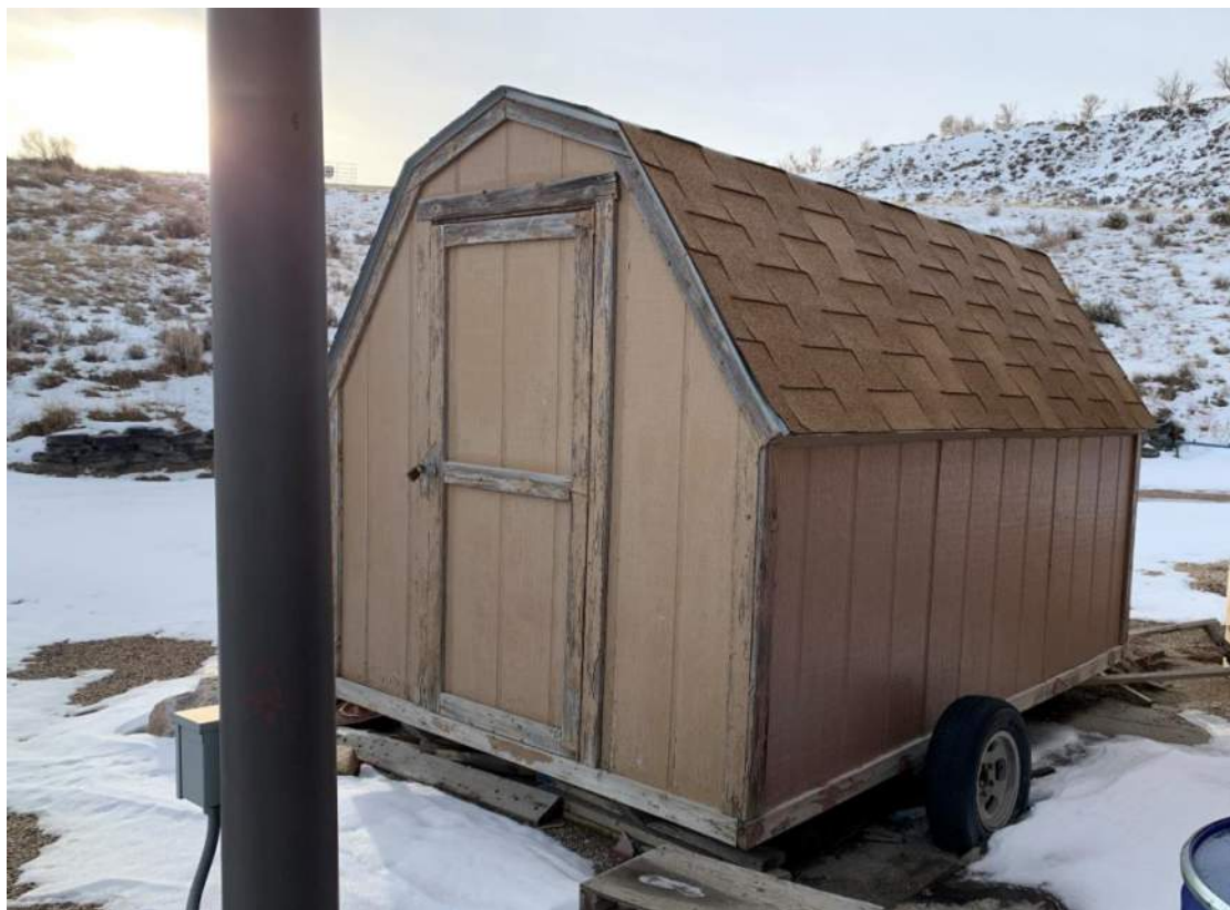
Storage Shed Adjacent to Firing Range Observation Tower
