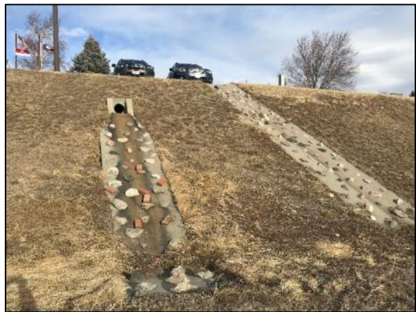
Drain Outlet and Curb Cut South of Visitor Parking
