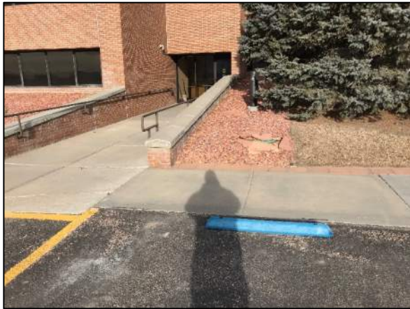
West Entrance from Visitor Parking Area
