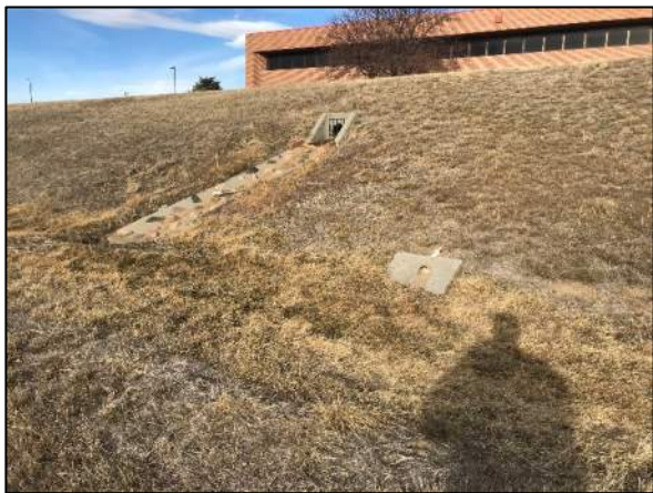
Drain Outlets South Side of WLEA
