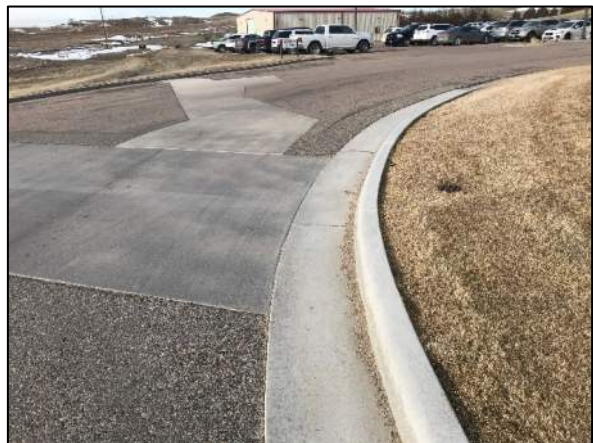
Drain Inlet Near Southwest Corner of WLEA
