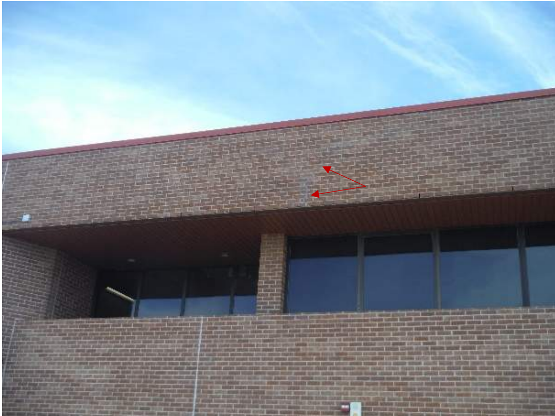
Area A - Repaired Cracks at West Upper Level Spandrel
