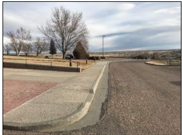
Pavement Near Main Entrance
