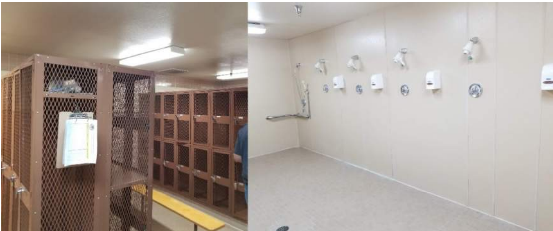
Existing Locker and Shower Facilities – Under-Utilized Space
