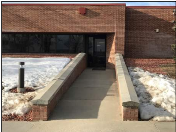
South Access from Staff Parking
