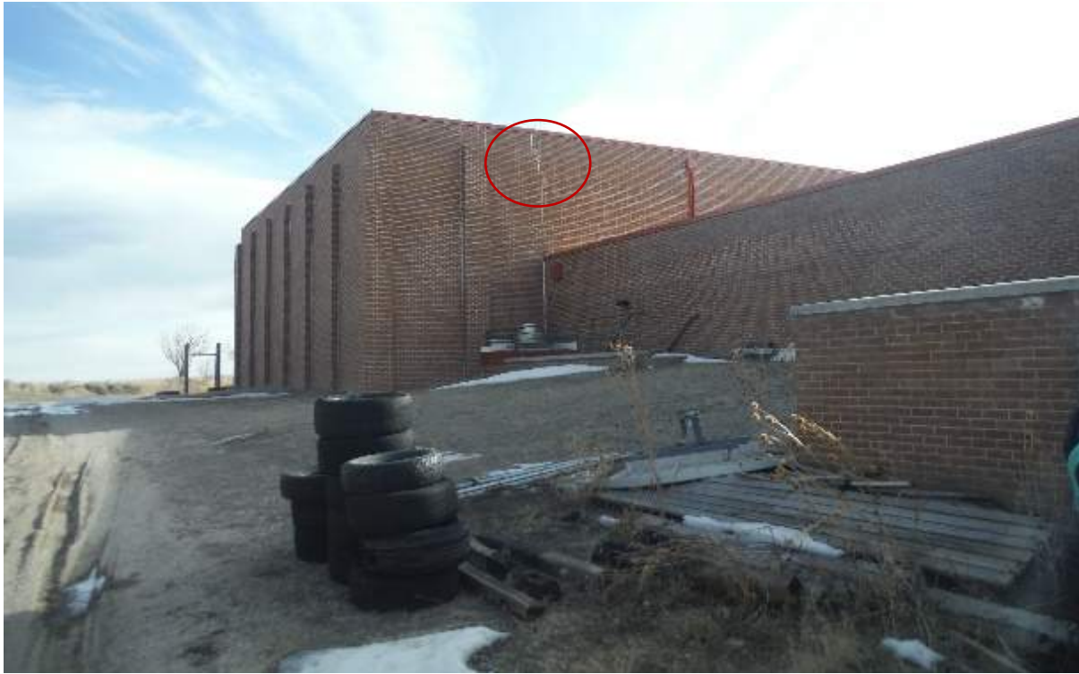
Area C - Repaired Cracks at Northwest Corner of Gym
