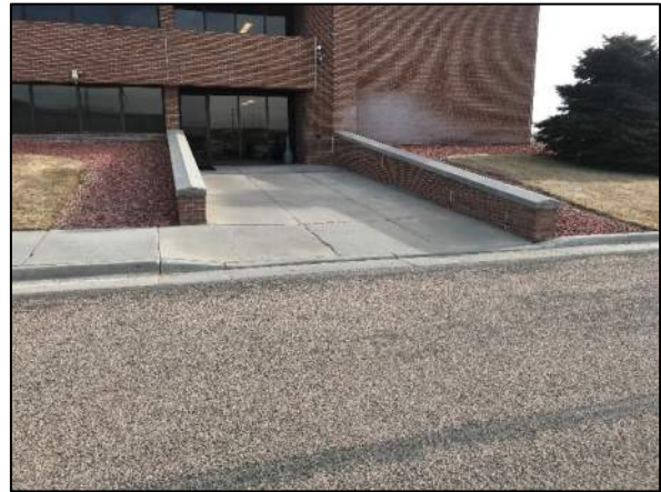
Southwest Entrance from Student Parking Area
