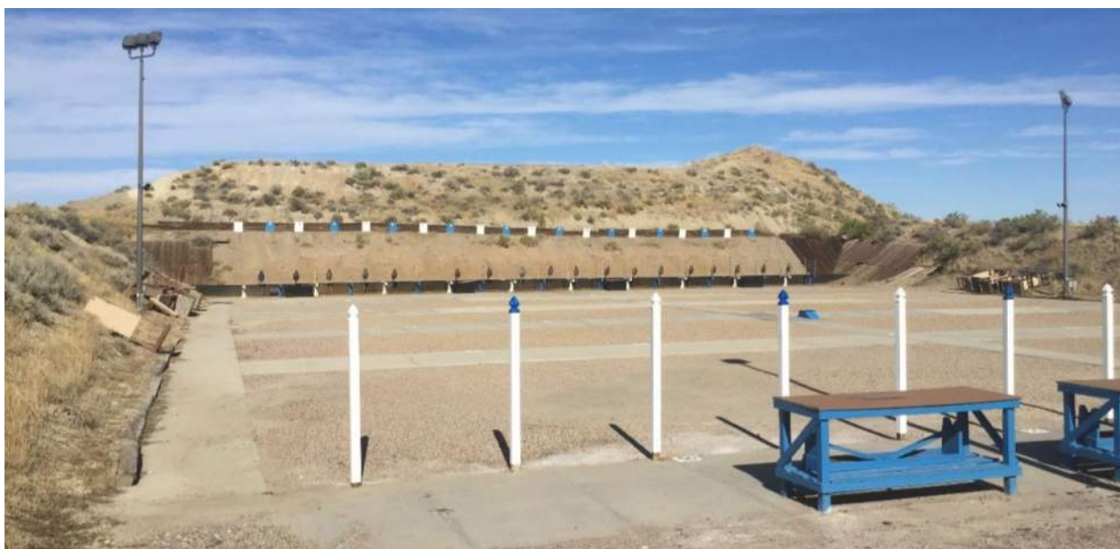
Outside Firing Range Line Stations and Backstop – Looking Northeast
