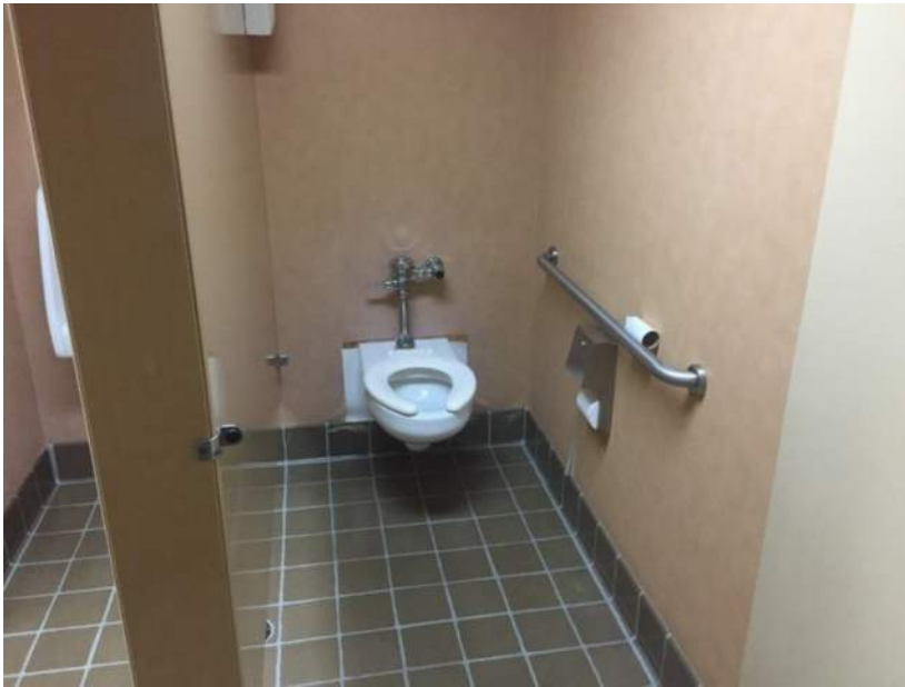
Public Restroom at Lobby Area
