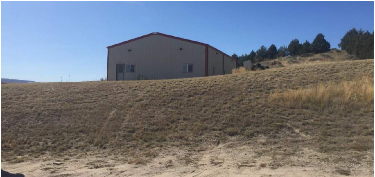
Maintenance Building as Viewed from Northwest Corner of the Main Building
