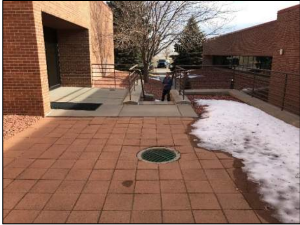
Drain Inlet in Courtyard South of Gymnasium
