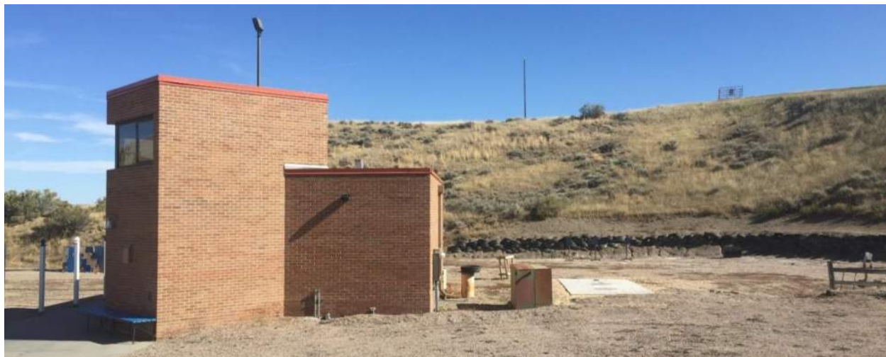
Observation Tower, Ready Room at Ground Level and Storage with Pistol Pit Behind (to the right in the photo)
