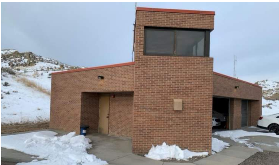
EVOC Observation Tower and Garage Bays Beyond
