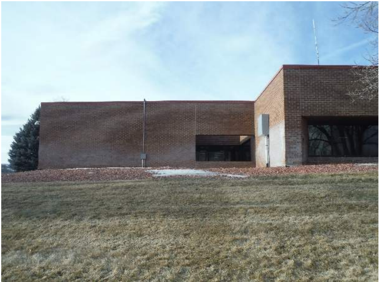
Area B - Southwest Corner
