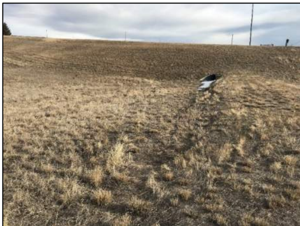
Embankment for North River Bend Road
