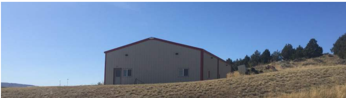
Existing Maintenance Building
