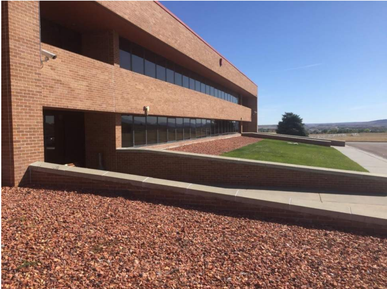
The Southwest Elevation of the Main Building at the Dormitory Area
