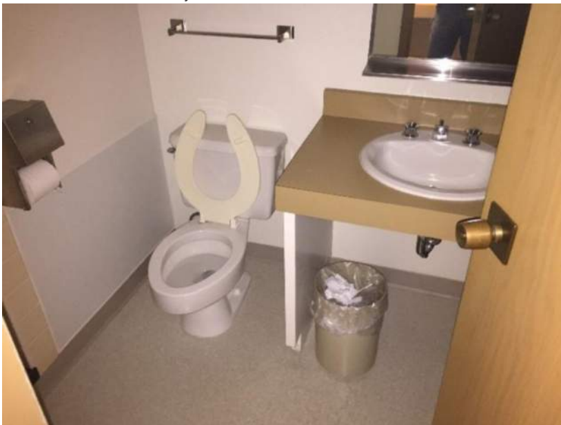
Restroom in Dormitory
